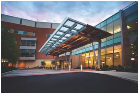
Figure 8. New Women & Infants' South Pavilion adjoining existing hospital.
